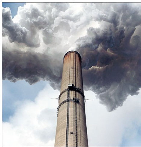
A North River Sewage Treatment Plant smokestack actively discharging. 22
